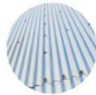
Profiled metal roof
