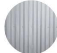
Profiled metal roof
