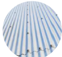
Profiled metal roof
